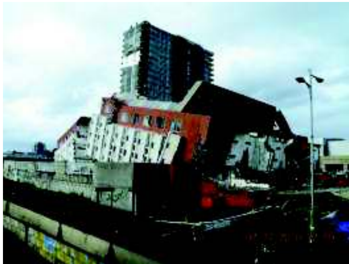
Figure 4. The collapsed Alto Rio apartment building in Concepción. Eight people were killed when this building fell over.
