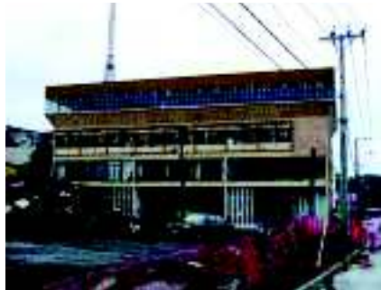
Figure 8. Damaged Firehouse in Talcahuano, near Concepción.
